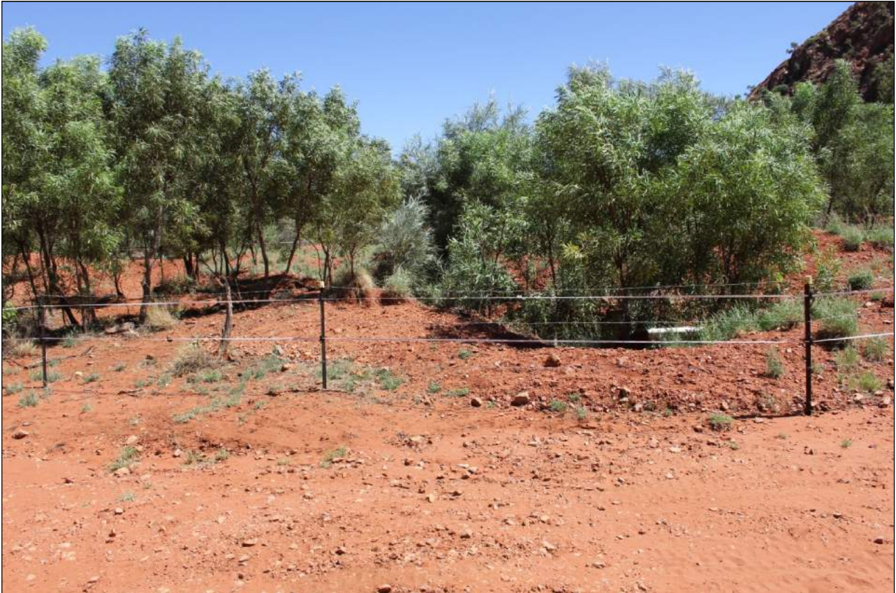
Figure 9. Photograph showing the fenced waste water evaporation sump. The fence is made up of a combined five tier barbed wire and low voltage portable electric fencing (white) to exclude stock.
