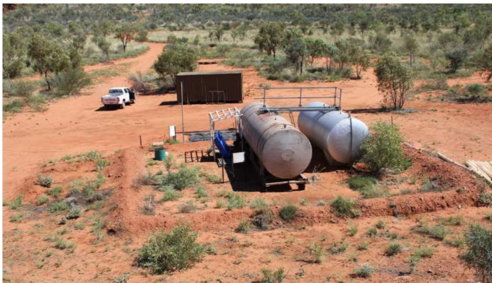
Figure 6. Fuel farm view looking north (2013) showing earthen bunds (the facility is not in use and will be replaced in the future).
